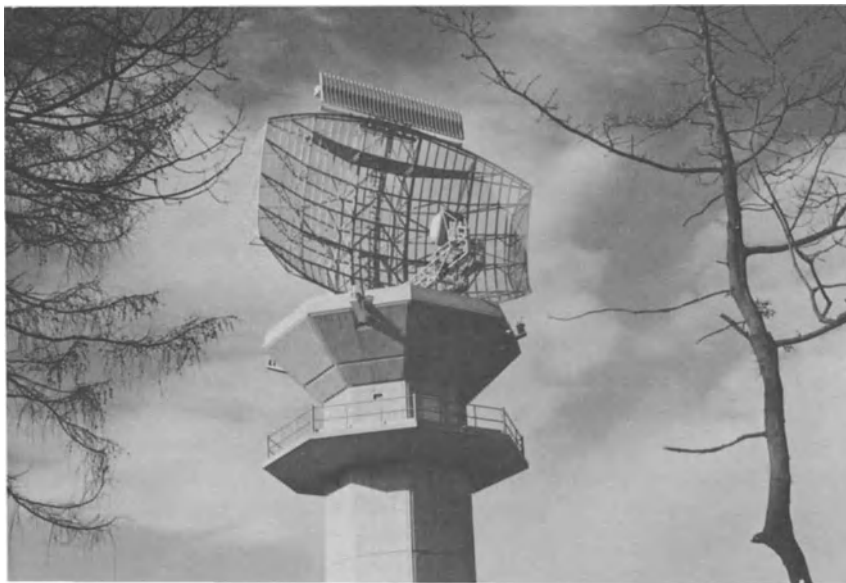
Figure 1.2 The antenna of a long-range radar used by the British Civil Aviation Authority for aircraft surveillance (photo: Paul A. Lynn)
